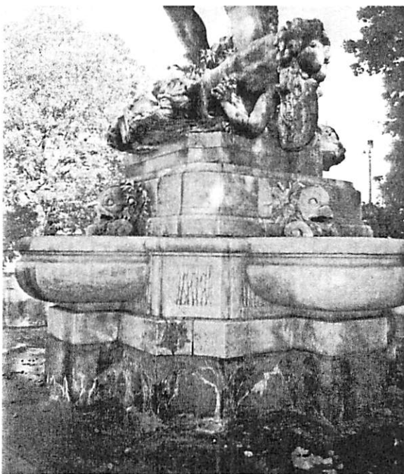
An example of the accumulative deterioration from general neglect, environmental and mechanical damage.
